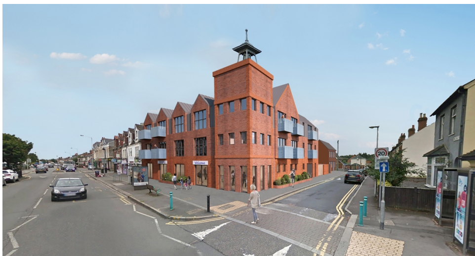
Balconies with glass
