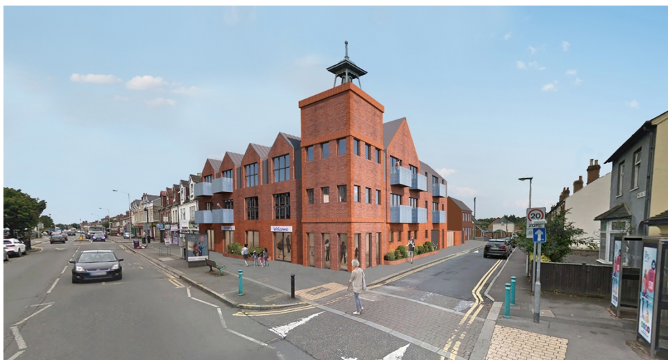
Balconies with glass
