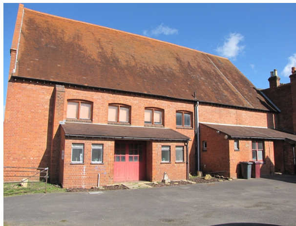
Rear elevation of church
