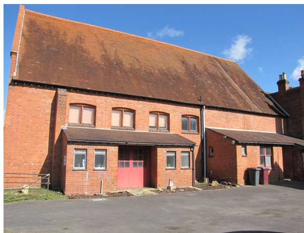
Rear elevation of church
