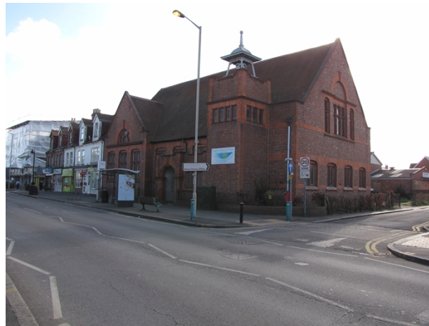
Photo taken from opposite side of Oxford Road of Wilson Road junction
